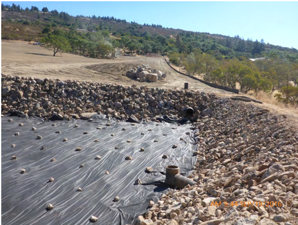
Photo 6. Photograph of detention basin.
