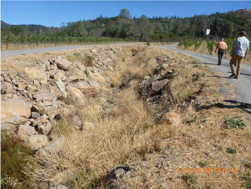
Photo 1. Lower portion of unnamed intermittent stream that was channelized (looking upstream).
